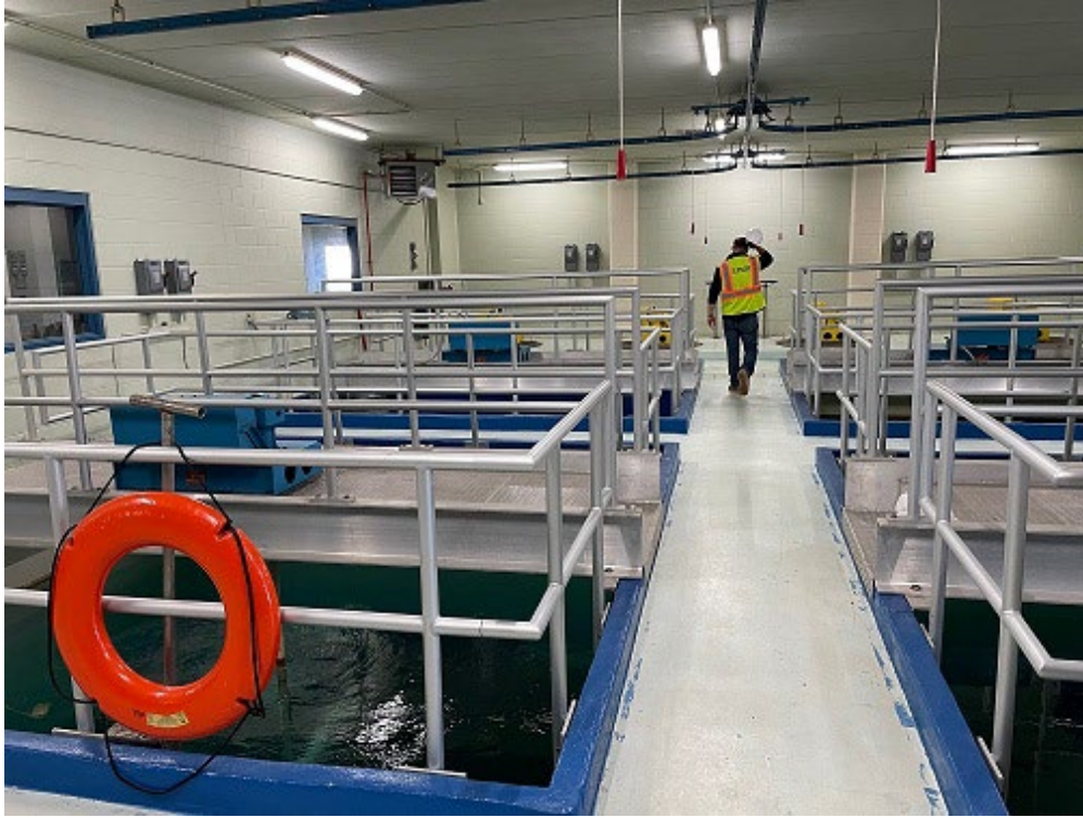
The flocculation basins(above) and filters (below) in Two Harbors.
