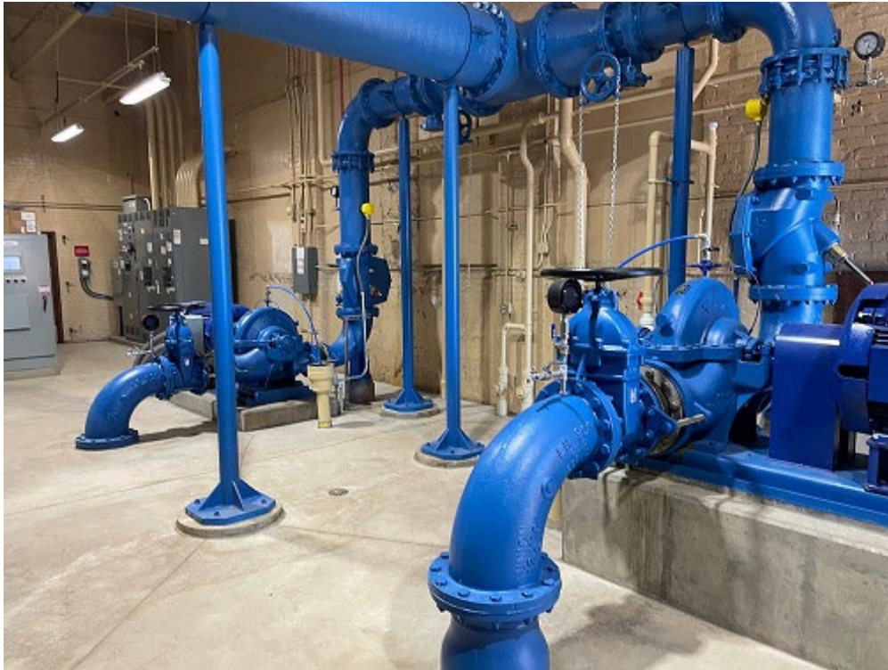
The pumps and surge tank in the Duluth booster station.
