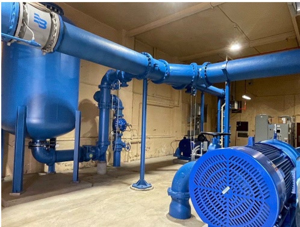
The pumps are on the same spots as the previous ones although the new pipes are underneath the building. Another change was the addition of a surge vessel with a bladder tank. Soderlund said
