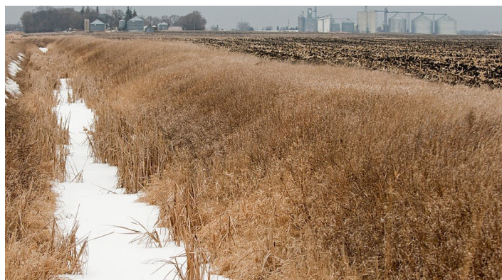
Drainage Ditch (Jackson Forderer, 2012)
